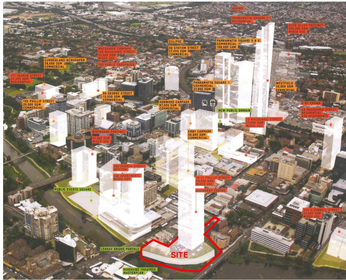
Figure 26 – Site context: changing nature of Parramatta CBD built form (source: Council - with site location added by JBA)
